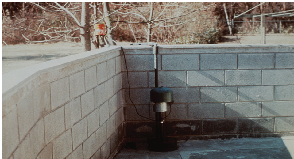
Figure 8-6. Small patio floodwall with sump pump.
